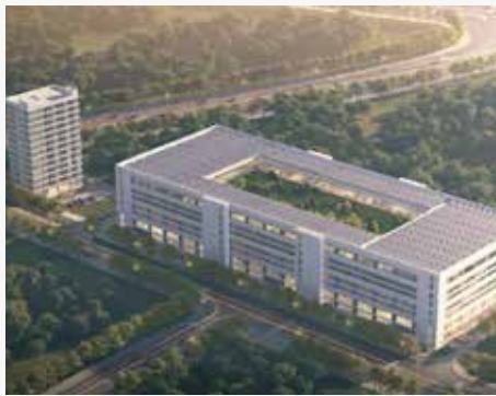
Guangdong Pipeline Production Base
